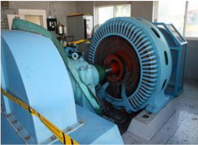
One of two hydro-electric generators at the Brigham City Power Plant visited by members of the Box Elder Chapter.
