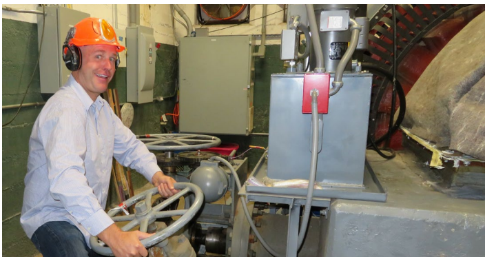
Jim Williams operating the valve controlling the 200 psi flow of Little Cottonwood Creek into the red turbine spinning at 400 rpm.
